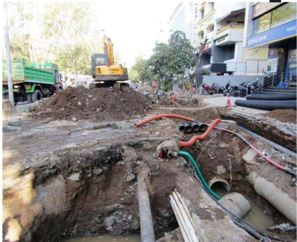
Fig. Complex network of existing underground utilities at different levels in DP Road, Pune
