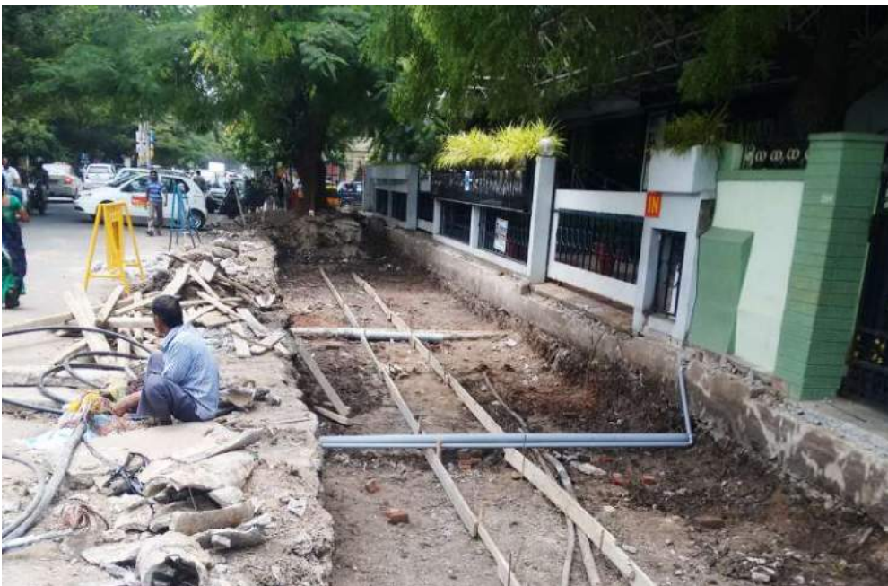
Fig. (above) Excavation work carried out in Coimbatore ahead of the rainy season to prevent stagnation of water
