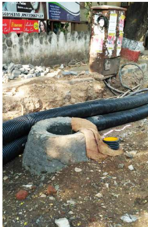
Fig. (top left) Multiple utility lines in one manhole due to lack of space in DP Road, Pune
