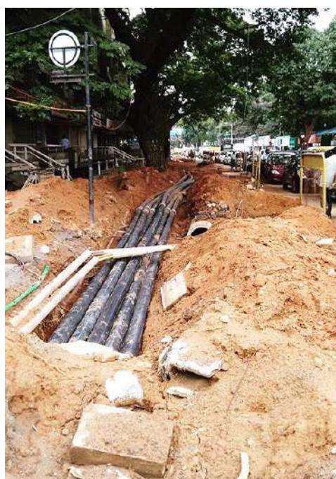
Fig. (left) Damage caused by excavating beyond 2 m around trees in Coimbatore
