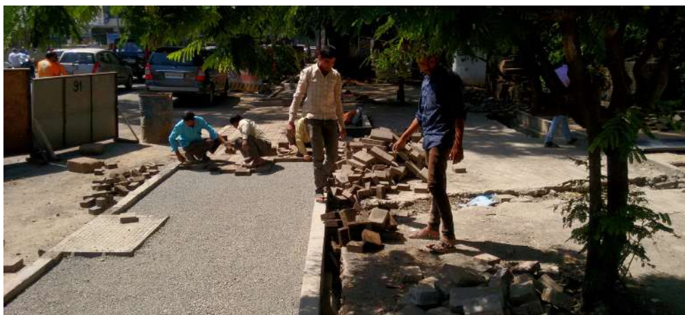
Fig. Paving tiles/blocks are laid on the compacted base to finish the footpath. This requires fine workmanship to ensure that the blocks are laid close together and do not come loose in the future.
