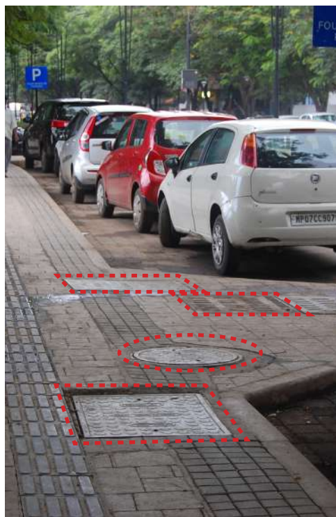
Fig. (top left) Manholes at bulbouts and utilities at tree pits in JM Road, Pune
